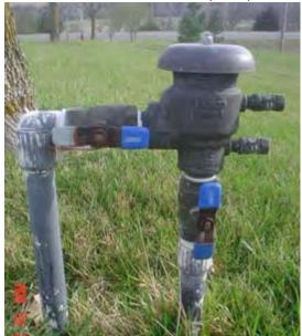
testable backflow preventers, PVBs have two shut-off valves.
