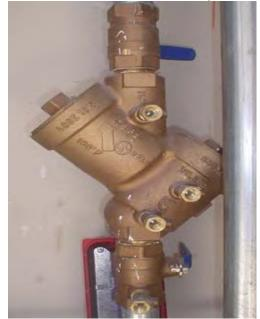
spring-loaded check valves sandwiched between two shut-off valves. A check valve is a one-way valve that will let water flow through it in the correct direction, but closes if water tries to go backwards. Think of it as a door you can exit through, but doesn't have a knob on the other side for you to get back in. There are two check valves on a DCVA, so if one fails, there is a back up.A shut-off valve is just what it says; it shuts off the water. It is like the
