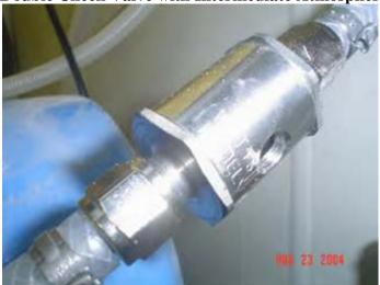
These are small devices used on post-mix carbonated beverage dispensers. The International Plumbing Code specifies that they be used for such applications, but City of Manhattan staff prefers RPZs, because they can be tested. In post-mix carbonated beverage machines, there is a danger of carbon dioxide or carbonated water backflowing into the water supply (see below). Double check valves with intermediate atmospheric vents work similar to an RPZ to prevent this from happening.
